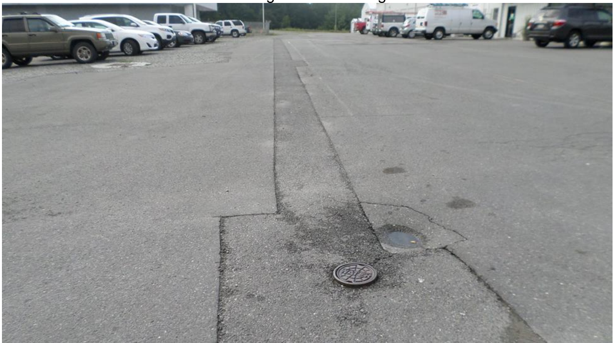
New Water Line
